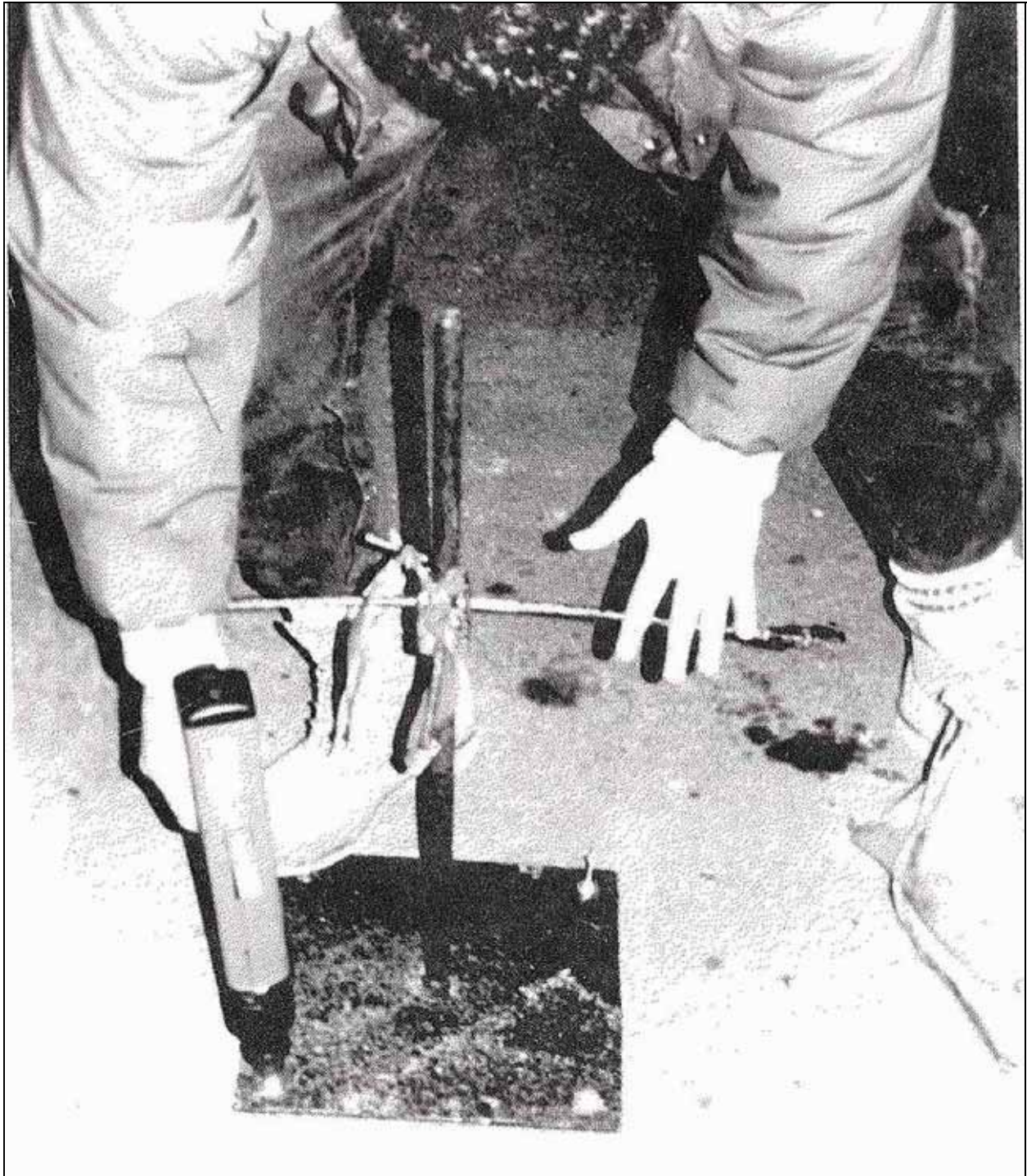
Figure 5. Setting an Erected Stringline
