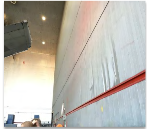
Figure 1: Damage on the Delta Air Lines hangar wall from wingtip collisions in Atlanta, GA
