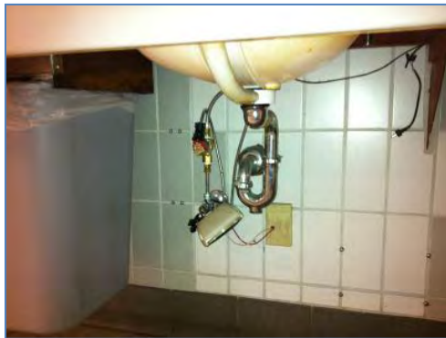
Figure 6: Damaged Restroom Plumbing
