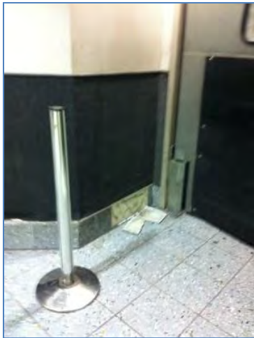
Figure 7: Damaged Wall Tiles
