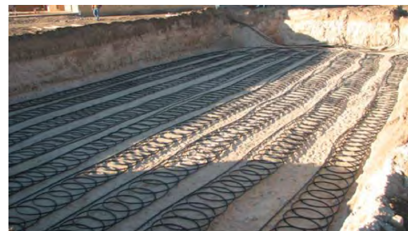
Figure 12: Horizontal slinky configuration
