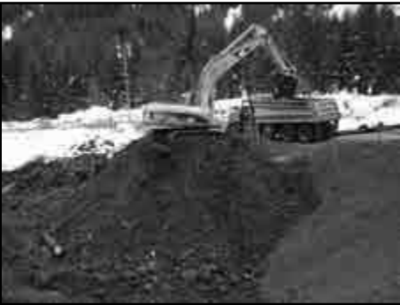
Figure 3. Removal of contaminated soil [9]
