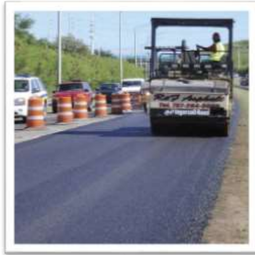
Figure 13 Rubberized asphalt being applied to a road (Asphalt Photograph, 2014)
