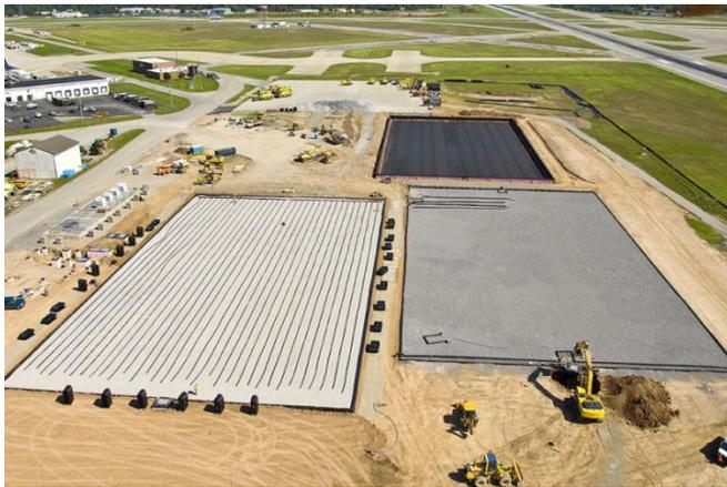
**Figure 1: Construction of aerated gravel beds at Buffalo-Niagara International Airport**
