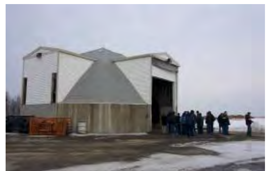
Figure 11 – Inspecting the Sand storage facility at BGM
