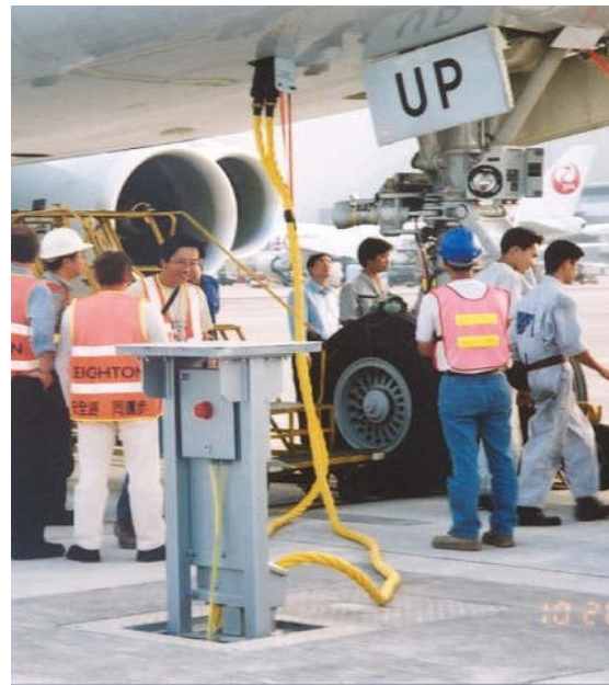
Figure 5. Pop-up 400Hz cables in Hong Kong (Ref: McFadyen)
