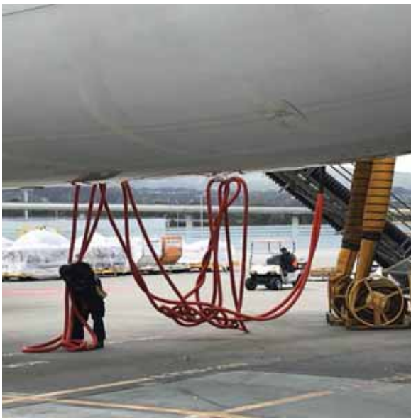
Figure 4. 400Hz cables at SFO
