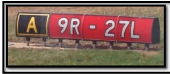
Figure 8 Mandatory Sign and Location Sign at The Ohio State University Airport
