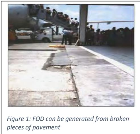
maintenance, and construction of the airport infrastructure can also contribute to FOD. According to Boeing, pieces of concrete can break loose from holes in pavement or from fatigue corner cracks and building materials can fall from construction vehicles or be blown from gate areas onto airplane maneuvering areas (Figure 1). Broken pieces of pavement can collect at the edge of the gate area and be
