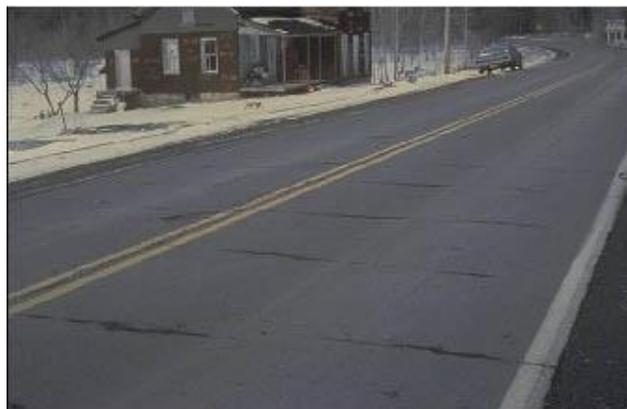
*Figure 5: Transverse cracks caused by thermal cracking in a roadway pavement.<sup>9</sup>*
