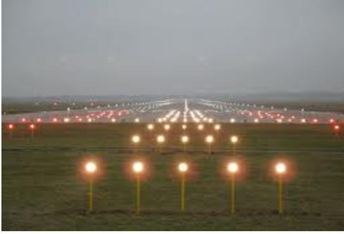
Figure 17 – A typical runway lighting system [45]
