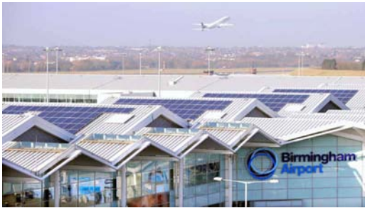
Figure 2 – Solar Panels on the roof of the Birmingham Airport [5]
