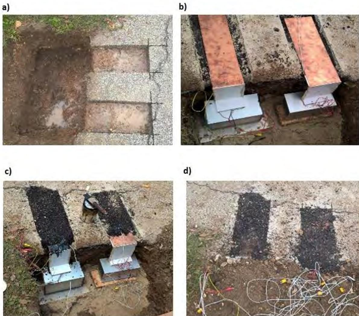
Then top surface of the heat conducting metal plate were covered with hot mix asphalt at to restore the road surface (Fig. 5.13c). Temperature sensor probe's wire including the TEGs wires were taken out to the soil surface before the pit is backfilled to the existing ground level (Fig 5.13
