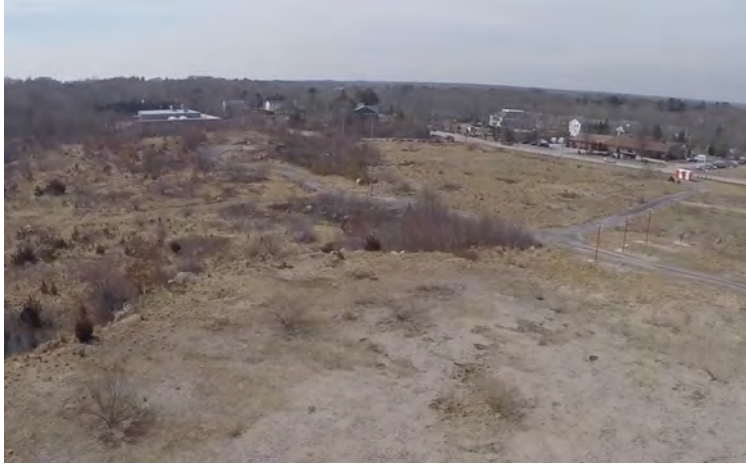
(a) Inaccessible area
