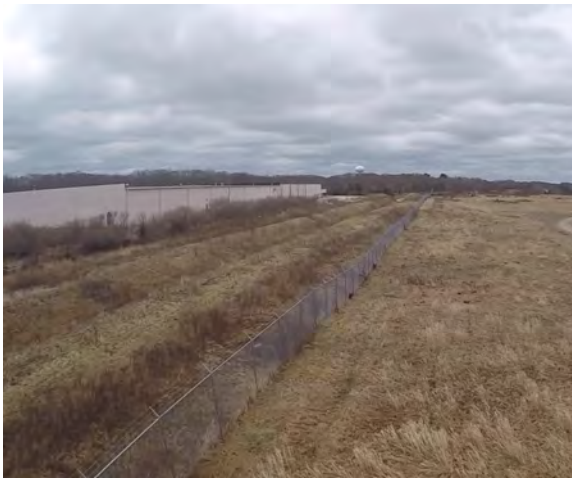
(a) Fence in perimeter inspection
